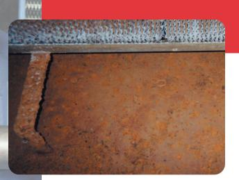
An HVAC unit's humidifier pan was corroding and in need of immediate attention.
