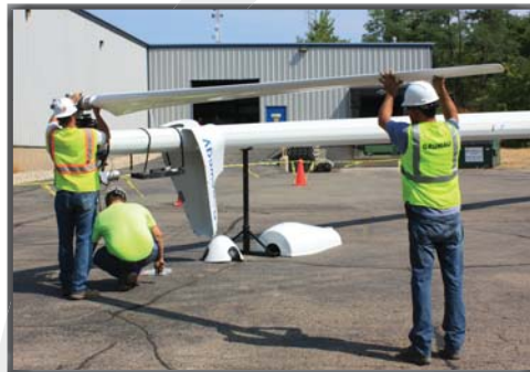
Attaching 1 of the 3 large turbine blades
