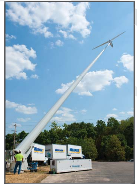
Erecting the assembled wind turbine and tower
