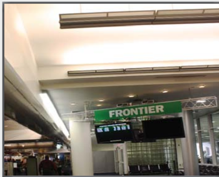
Grunau-installed energy-efficient lights span the airport ticketing area
