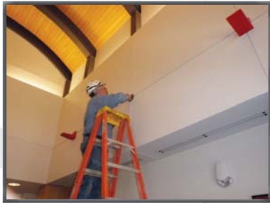
Grunau electrician installing energy-saving lights in office lobby
