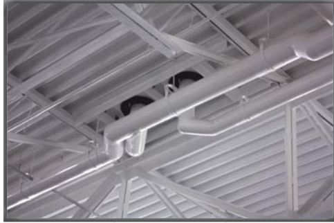
Hangers holding pipe on ceiling
