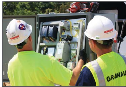
◀ Grunau Electrical Team installing and finalizing the electric control system at base of wind turbine
