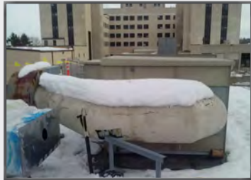
Before the remodel
