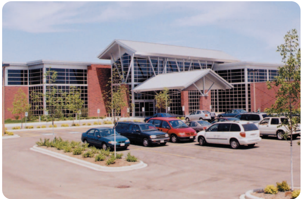
The Grunau team worked above and around the existing Advance Healthcare facility in Mequon to complete the design/build of a surgical suite addition.
