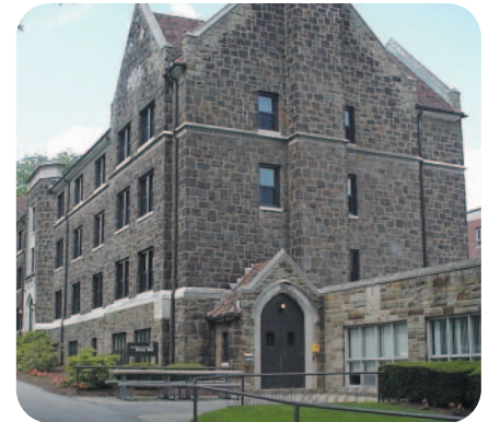
The Youngstown fire protection office retrofitted wet and dry sprinkler systems for three Westminster College dormitories, including Browne Hall. Built in 1957, the hall houses 108 female students.
