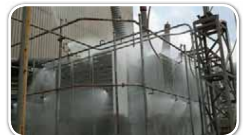
▲ A fire protection discharge test is run at Sammis after the emergency installation of a new transformer.
