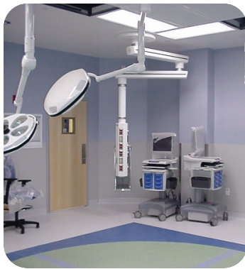
◀ Grunau’s dry fire protection system will help protect sensitive equipment in Humility of Mary hospital operating rooms.
