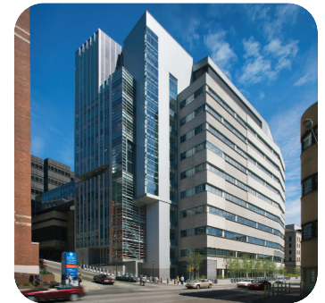
▲ Grunau’s technicians installed the fire protection system for BST3, the new biomedical science building at the University of Pittsburgh.
