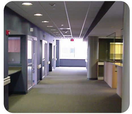
▲ Grunau installed the fire protection system for the newly-constructed Humility of Mary hospital.
