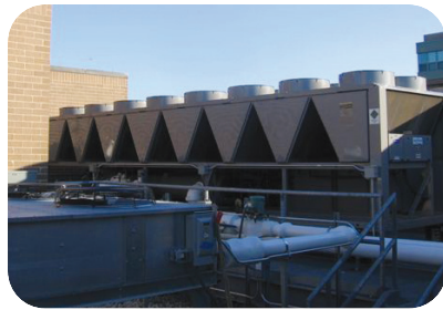
▲ At the Jewish Home and Care Center in Milwaukee, Grunau installed part of the HVAC system on the roof due to the obstructions around the building.
