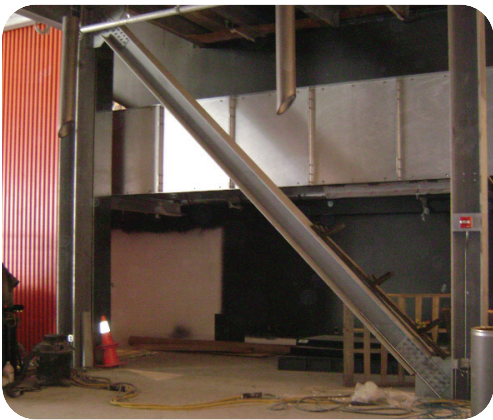
◀ Grunau's metals technicians fabricated and mounted the support steel on the interior of the Harley Davidson Museum in Milwaukee.
