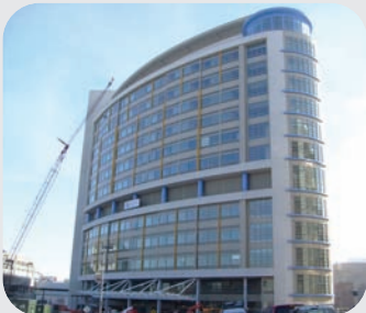
▲ Grunau managed plumbing installations for the new 168-room bed tower at Children's Hospital of Wisconsin.
