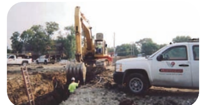
▲ The Grunau team needed to dig trenches for piping that connected to geothermal wells at Johnson Controls.
