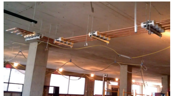
Quickly installed at the jobsite
