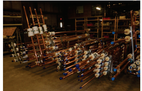
Prefabricated in Grunau's shop
