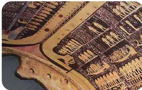
Grunau carefully placed camouflaged sprinkler heads in the ceiling of the “Revenge of the Mummy” amusement park ride to blend in with the attraction's hieroglyphics.
