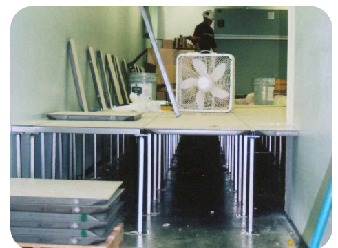
To allow room for an underfloor HVAC system, piping and computer wiring, Grunau's service and maintenance team oversaw the installation of a raised floor for Aurora Health Care's second computer room expansion.
