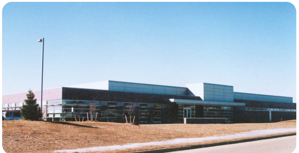
Grunau recently completed mechanical, plumbing and fire protection work on a building for Thomson BETA Systems. Headquartered in Milwaukee, Thomson BETA is one of the largest data-processing firms in the country.
