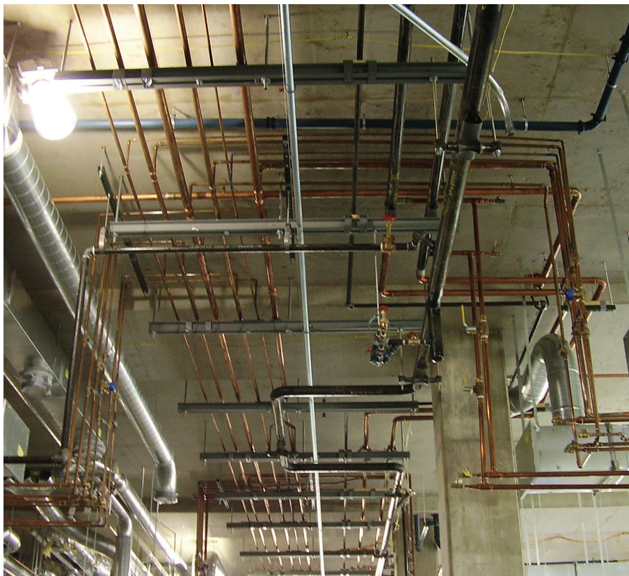
Coordination was a key issue for contractors on the Biomedical Research Building project in part because of the extreme amount of piping runs in the facility.
