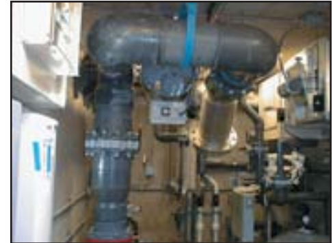
Typical Pump Vault
