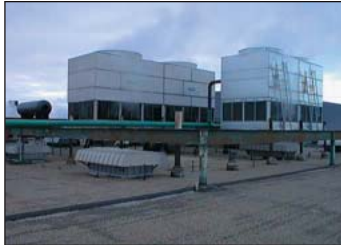
Cooling Towers – Structural Steel & Piping
