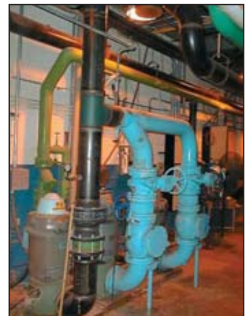
Modification to Pumps & Piping
