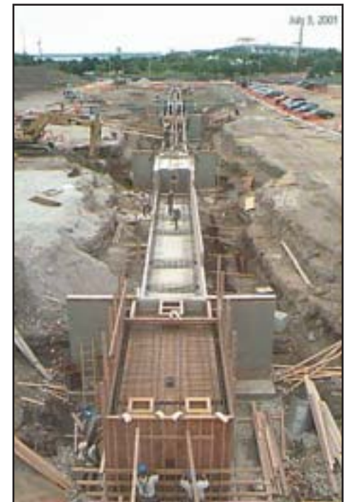
Pump Vaults, Water-Well Structures Under Construction
