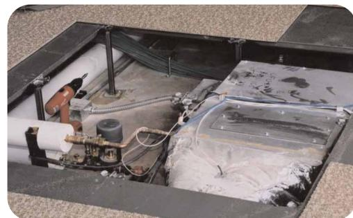
*The Grunau mechanical team installed an underfloor HVAC system, placing the heating and cooling vents under a raised floor instead of above the ceiling like a standard overhead unit.*
