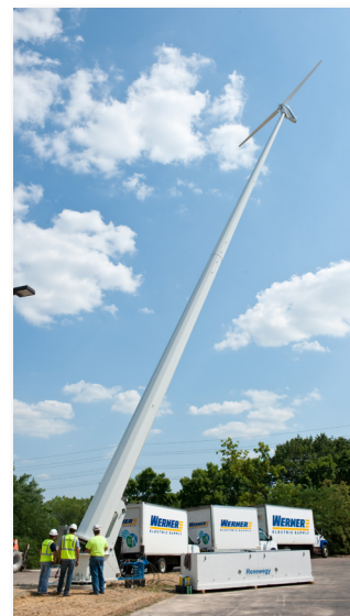
Erecting the assembled wind turbine & tower
