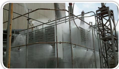
▲ A fire protection discharge test is run at Sammis after the emergency installation of a new transformer.
