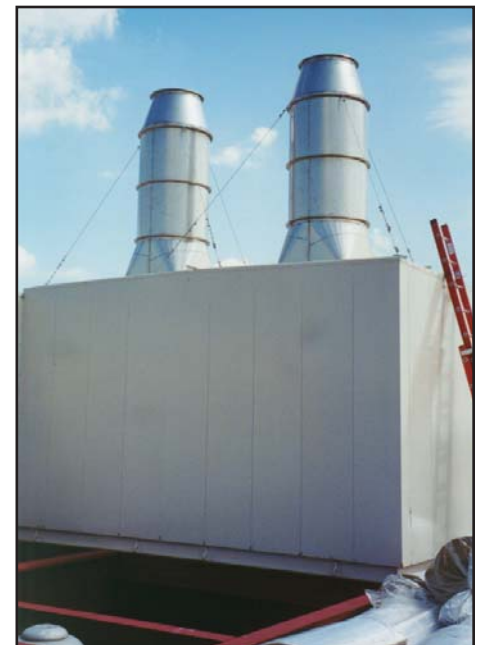
Lab Hood Exhaust Stacks
