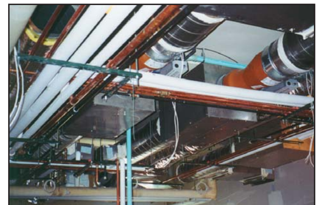
Overhead Mechanical Services for Lab Hoods & Tables
