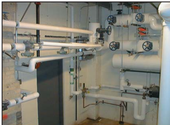
Steam Service Room
