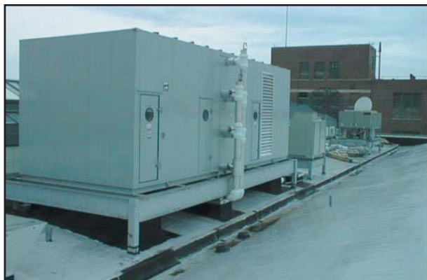
Custom Air Handling Unit & Chillers
