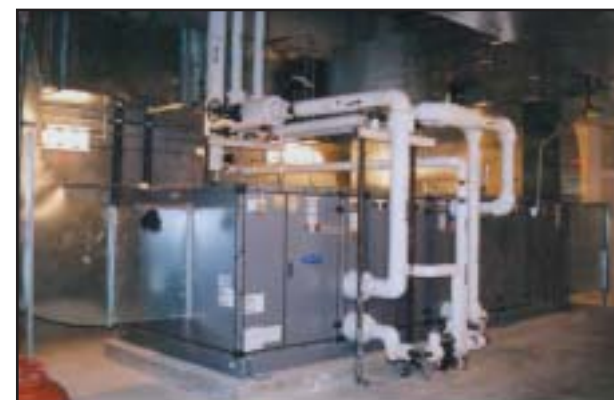
Typical Air Handling Unit
