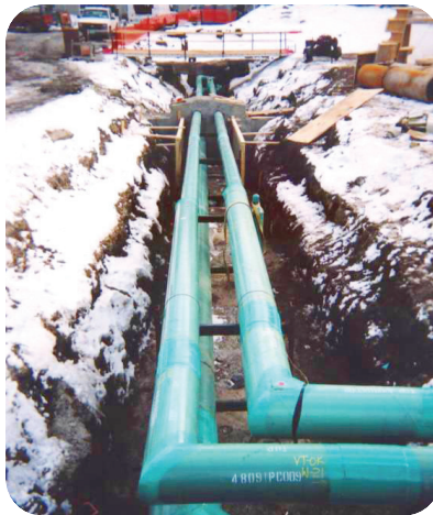
▲ Grunau's mechanical team battled the winter weather to reroute steam and pressure piping at the Medical College of Wisconsin's new $110 million research center.
