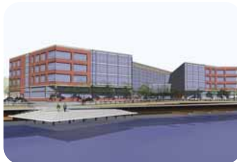
At Manpower's new headquarters Grunau Company installed HVAC, plumbing and fire protection systems, as well as miscellaneous metals.
