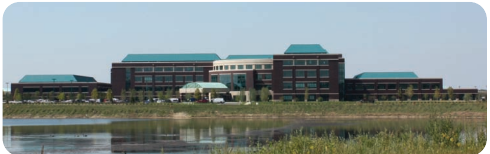
▲ Grunau recently completed plumbing and HVAC work on Aurora's new 800,000 square-foot hospital located in the town of Summit, Wisconsin.
