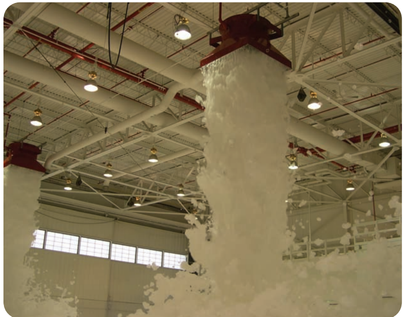
▲ Grunau tested its newly-installed high expansion foam systems during a fire protection upgrade at the 128th Air Refueling Wing.
