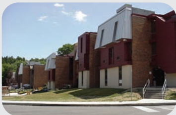
▲ Grunau's Pittsburgh fire protection branch installed new sprinkler systems in these student dorms at Robert Morris University and in two dorms at Duquesne University.
