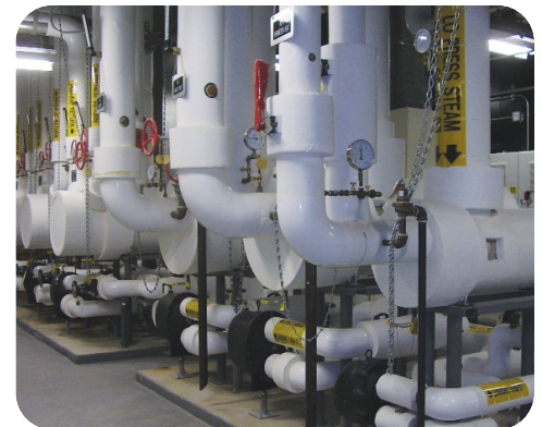
▲ The Grunau mechanical team installed steam-to-water heat exchangers that provide hot water to heat the building and reclaim heat from the exhaust air handling units.
