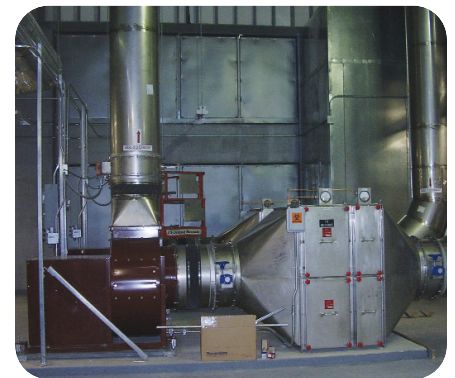
▲ A HEPA filtering unit cleans exhaust air from the vivarium biocontainment area in the basement of the Medical College of Wisconsin Research Center so that it can be safely released into the atmosphere.
