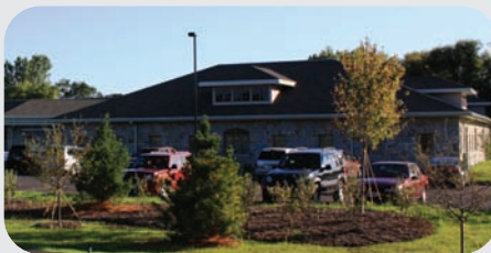
▲ Aurora Advanced Healthcare relied on Grunau for HVAC, plumbing and fire protection in its new Grafton clinic.
