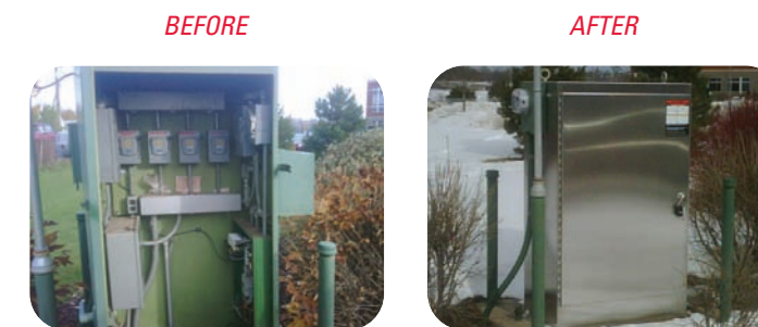
▲ City of Milwaukee Meter Pit
