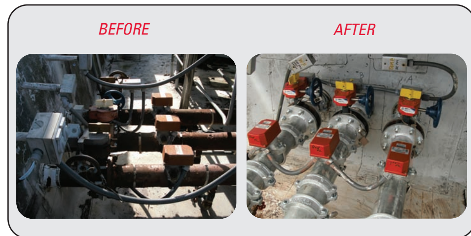
▲ Grunau's fire protection office in Orlando, Fla. replaced corroded fire protection equipment on the roof of Disney's Port Orleans hotel.
