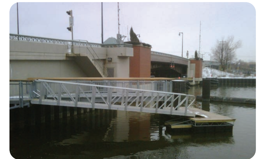
▲ The Grunau Metals team worked over water during the installation of this kayak dock along the Milwaukee River.
